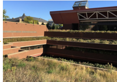
CIVIL ENGINEERING BUILDING
